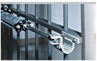
Operator shaft fixed to the gate
